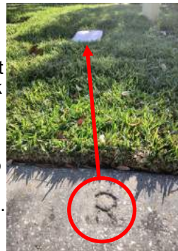
Above: burst 1” pipe past the valve box. Ran for hours until the valve cover was located and valve shut off. To find your valve, look for the R on the curb and follow it into your yard approx. 6-8 feet from curb. Right: R stamped into curb and corresponding exposed valve cover in grass. This is ideal for access.
