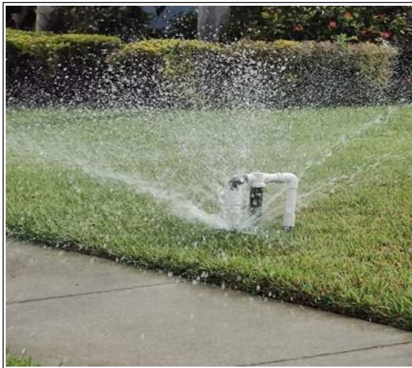
Above: burst 1” pipe past the valve box. Ran for hours until the valve cover was located and valve shut off. To find your valve, look for the R on the curb and follow it into your yard approx. 6-8 feet from curb. Right: R stamped into curb and corresponding exposed valve cover in grass. This is ideal for access.
